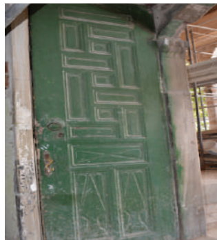
Figure 7. Main Door Wooden Wing
