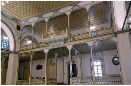
Figure 10. Sultan Murad Mosque Women's Section (Situation After Restoration)
