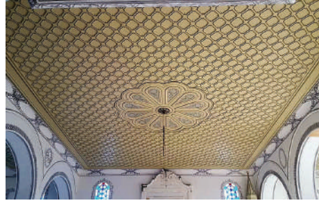
Figure 9. Harim's Sliced Wooden Ceiling (After Restoration)
