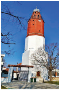
Figure 23. Skopje Clock Tower
