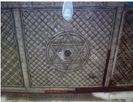
Figure 6. The Suleiman Signature in Wooden Ceiling
